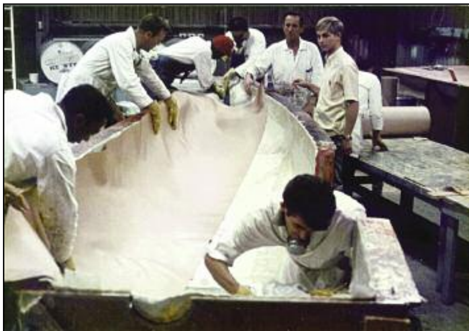
Dr. Leo and Ted Windecker inspected work on a half fuselage made of composites during construction of their Eagle. They are right rear with Ted in the yellow shirt. Two halves of the fuselage were molded separately and then glued together like a model airplane. Photo courtesy of Ted Windecker
